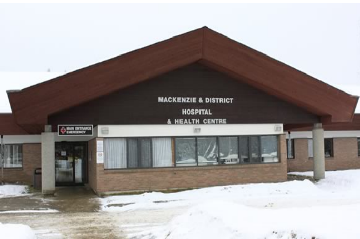
Photo above: Mackenzie and District Hospital & Health Centre
